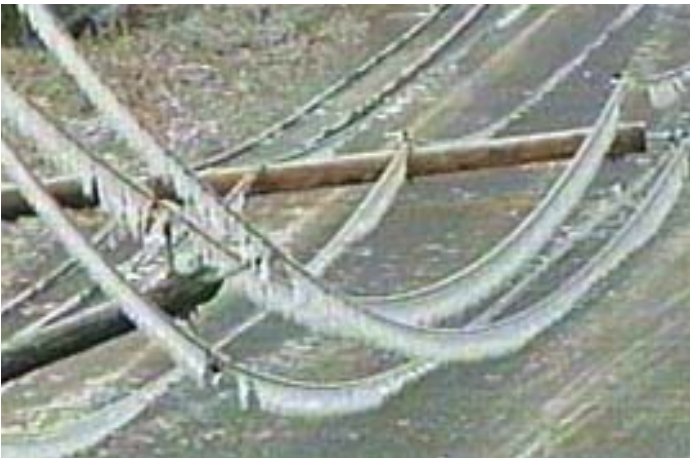
Ice Storm Damage
